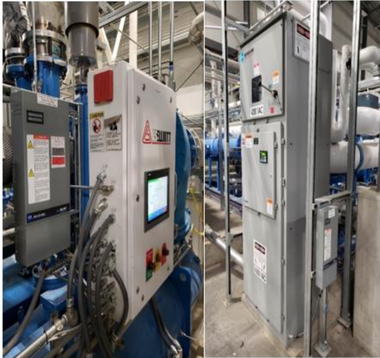
FIGURE 29: MiniDySC installation on LPCA-3.
