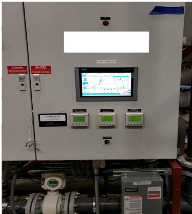
FIGURE 30: MiniDySC installation on RO skid.
