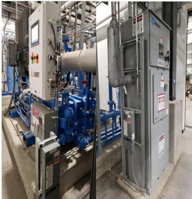
FIGURE 28: MiniDySC installation on HPCA-3.
